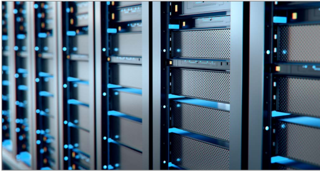
Setup for continuous automated testing
